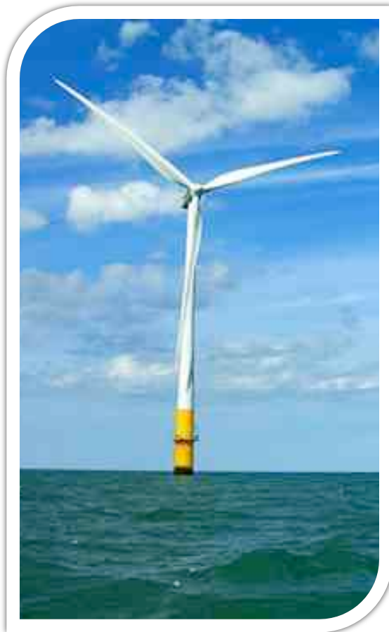
GE 3600kW Wind Turbine
