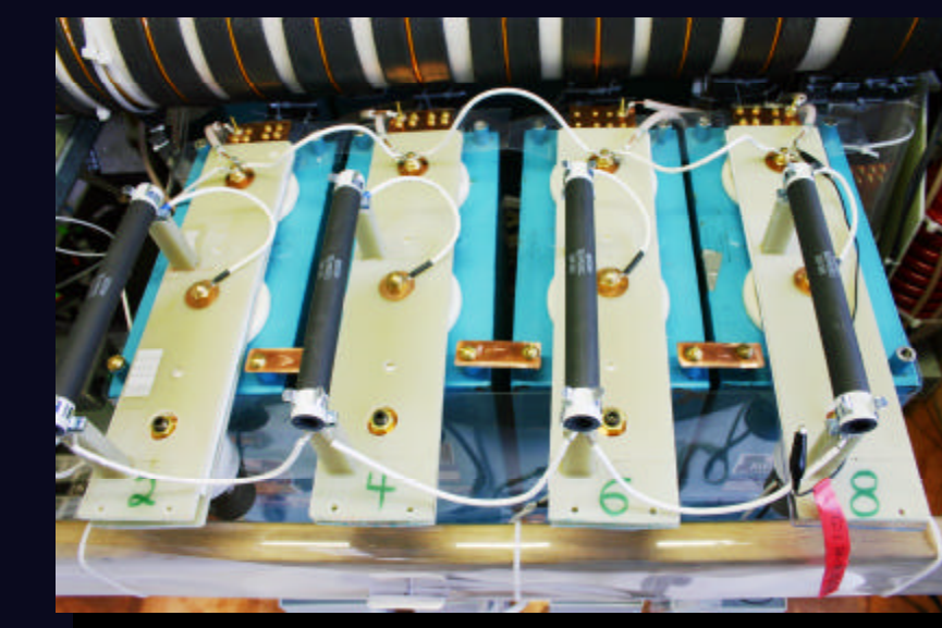
25kV, 14 uF capacitors
